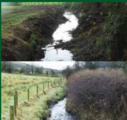
Eroded bank exposing sediment before fencing & after fencing vegetation regrowth ©VickyVeerkamp, DKIT
